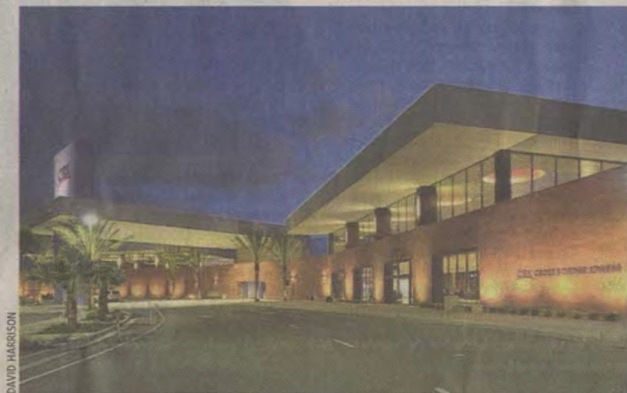
Cross Border Xpress resembles a typical new airport terminal. But it's a bridge in San Diego that speeds travelers to Tijuana International Airport.
